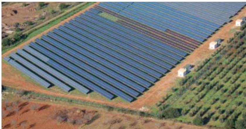
Solar plant developed by Madrilean company Affirma.
