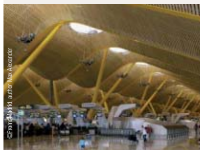
The new Terminal 4 at Madrid-Barajas airport.
