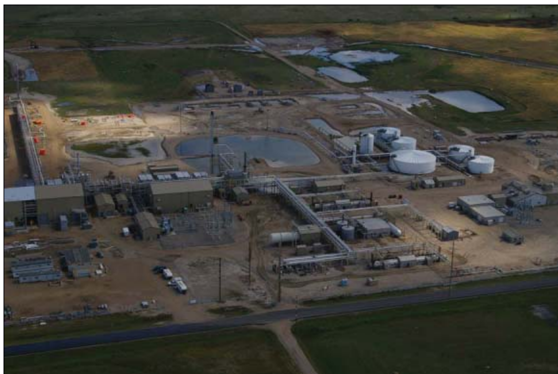
The Weyburn tank battery in Saskatchewan processes injected and produced fluids including CO 2 injected for enhancing oil recovery (Fig. 1)
