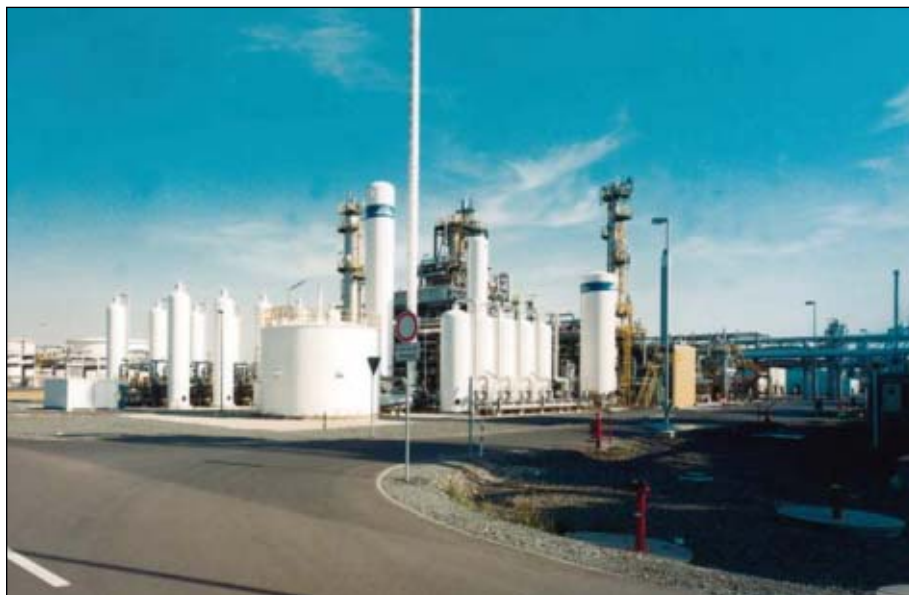
This PSA hydrogen plant is at the Leuna refinery in Germany (Fig. 2).
